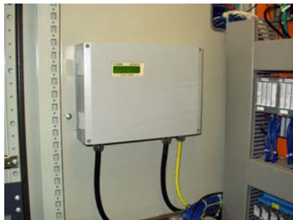
The transmitter FLUXUS ® ADM 7407 measures and controls the flow reliably.
