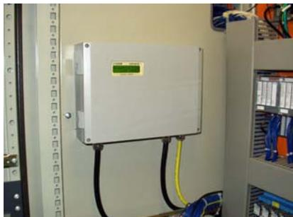
*The transmitter FLUXUS<sup>®</sup> ADM 7407 measures and controls the flow reliably.*
