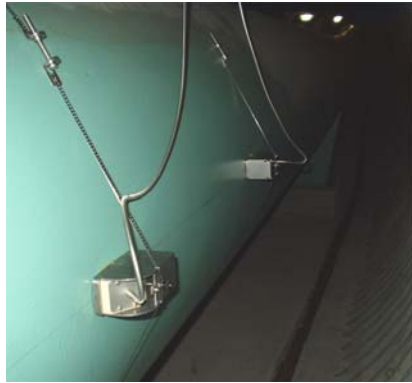
The alternative to costly underground construction and expensive inline measuring equipment: A non-intrusive flow measurement using the ultrasonic clamp-on procedure.
