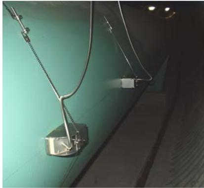
*The alternative to costly underground construction and expensive inline measuring equipment: A non-intrusive flow measurement using the ultrasonic clamp-on procedure.*
