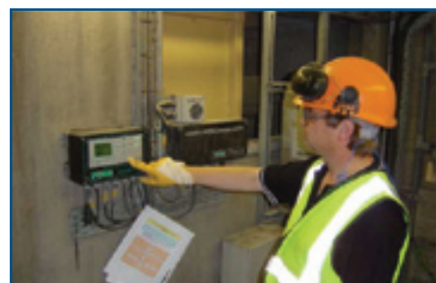
PCME systems allow the safe examination of the filter either at the control unit or remotely via a PC
