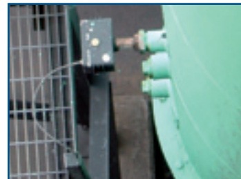
Pro-Scatter and Electrodynamic Main Stack Sensors
