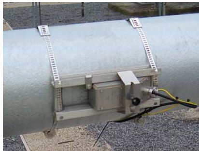
Stable fixation of the clamp-on ultrasonic transducers in the Variofix rail
