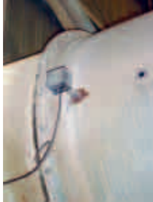
Electrodynamic DT system after bauxite crushing plant
