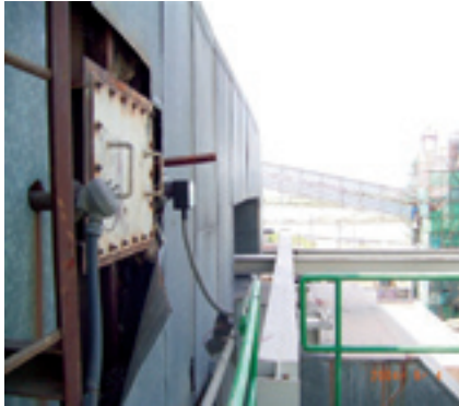
Accredited Dynamic Opacity instrument monitoring Electro filters
