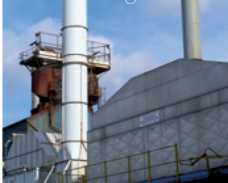
Emissions at hot rolling line can be monitored by PCME Electrodynamic Systems
