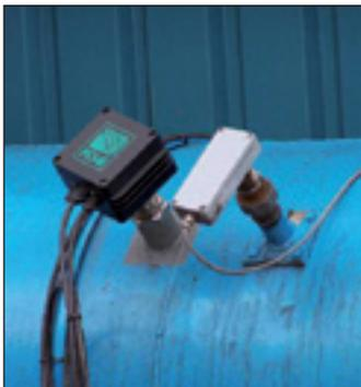
*A fully MCERTS approved Electrodynamic® instrument replaces non-compliant DC unit on Knockout Sand Plant.*
