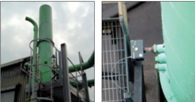
*Bag house on a Sand Plant monitored by an advanced Electrodynamic® instrument*
