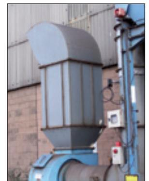
Networked Electrodynamic® Sensor used to remotely pinpoint bag row failure on a moulding sand plant
