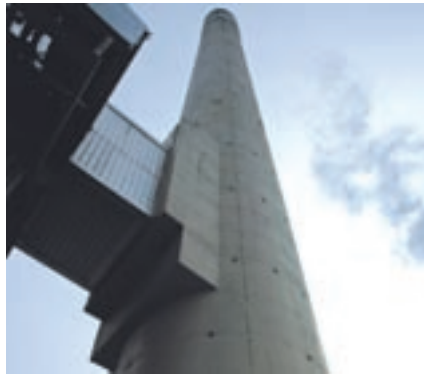
Kiln stack and electrofilter monitored by Dynamic Opacity instrumentation
