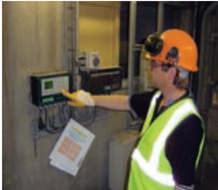
Filter condition assessed remotely
